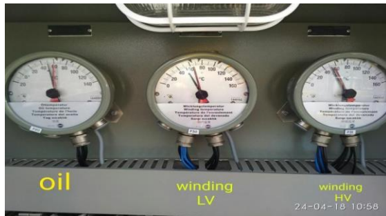
Gambar 3 Temperature Oil dan Winding
