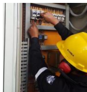
Gambar 12 Proses memasang kabel power supply
