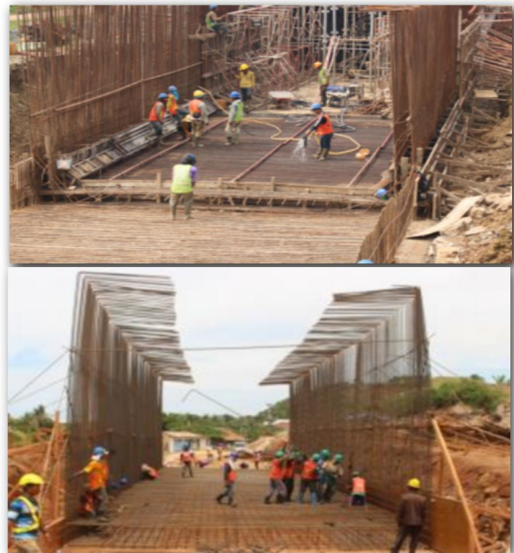
Gambar 3. Pekerjaan Pembesian & Bekisting Bottom Slab Box Culvert
