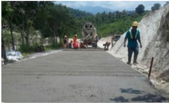
Gambar 2. Pekerjaan Cor Lean Concrete
